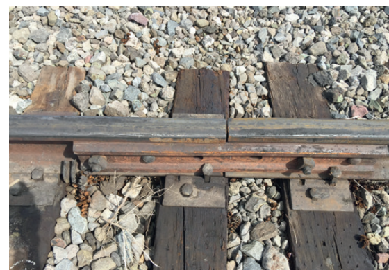
FIG. 6: The analysis of changes in rail joints supports the development of sustainable maintenance strategies
